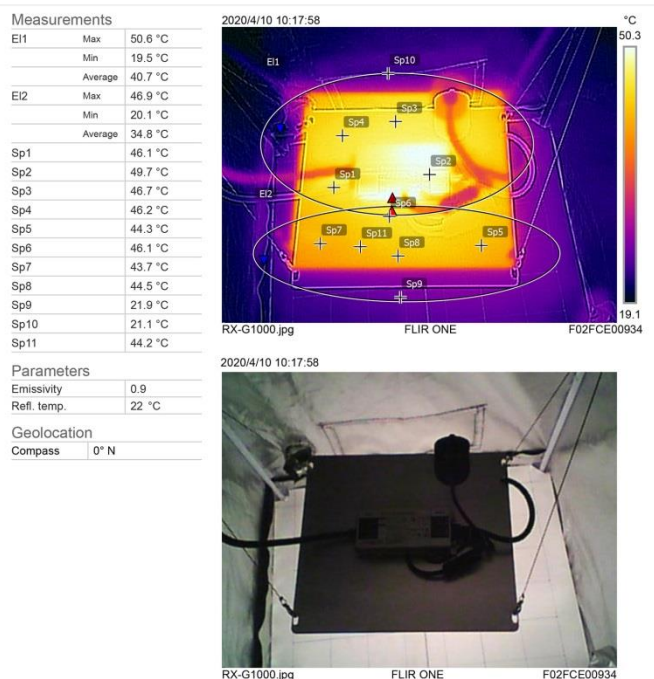
RX-G1000-SFI000 Surface temperature Test
